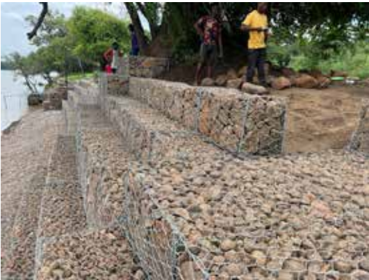
Supply of gabion boxes to Uganda Victoria Nile
