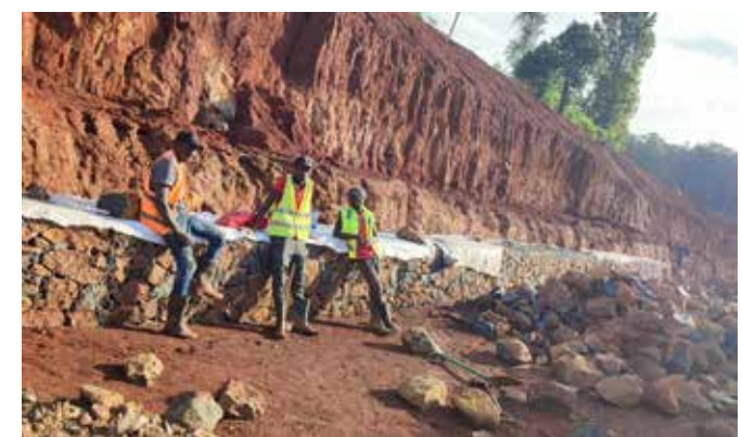
Supply of gabion boxes to Thika Rd, Kabati, Embu road construction
